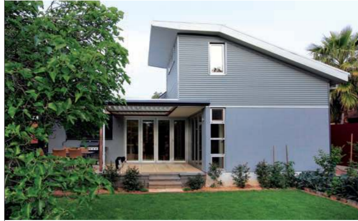
Retaining the original facade is a bold design element born out of a desire to add an element of surprise to an otherwise functional family home. The bluestone wall is coated in a specially designed membrane that helps regulate the temperature of the home throughout the year.
